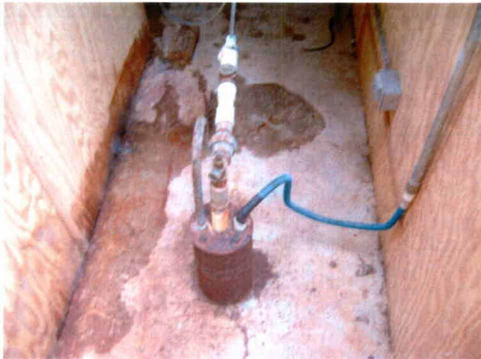
Photograph 2: View of the steel casing of the well.
