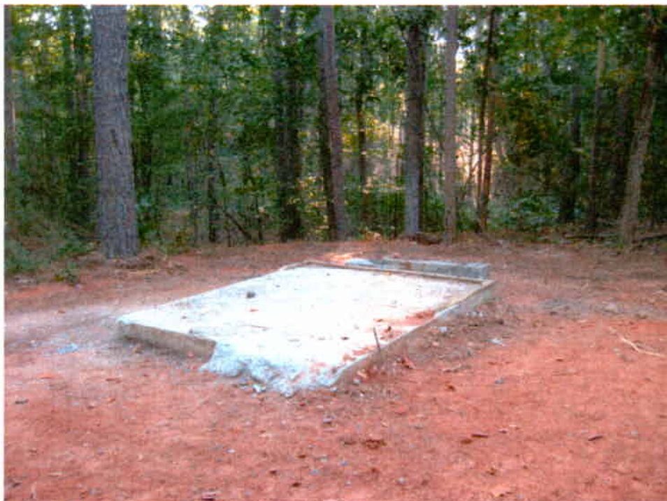
Photograph 8: View of the area after abandonment activities completed
