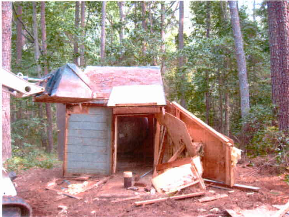
Photograph 5: Removal of the Well House
