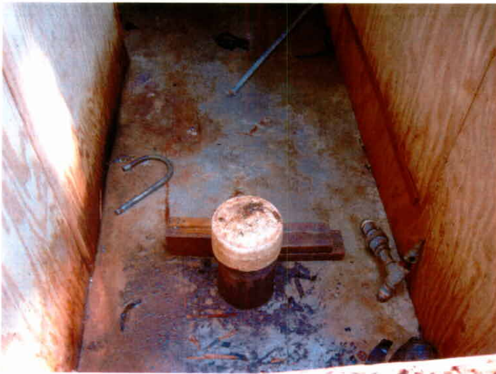
Photograph 4: View of the well sealed prior to demolition.
