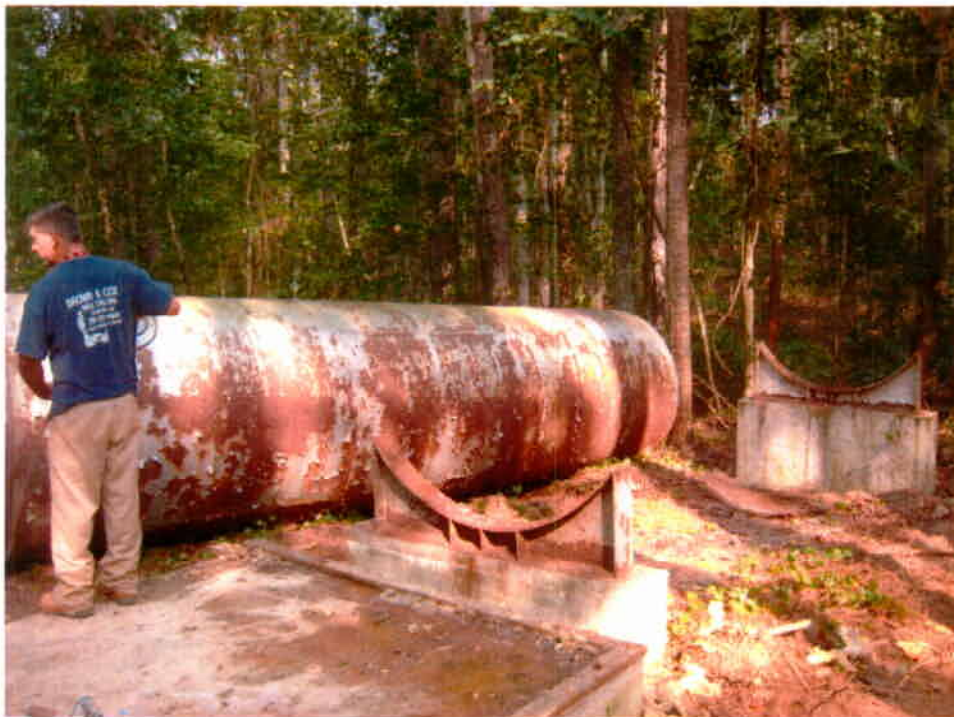
Photograph 6: Removal of the AST
