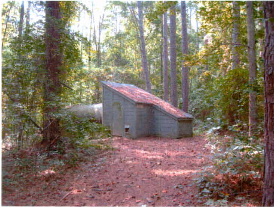
Photograph 1: View of Supply Well House and AST.
