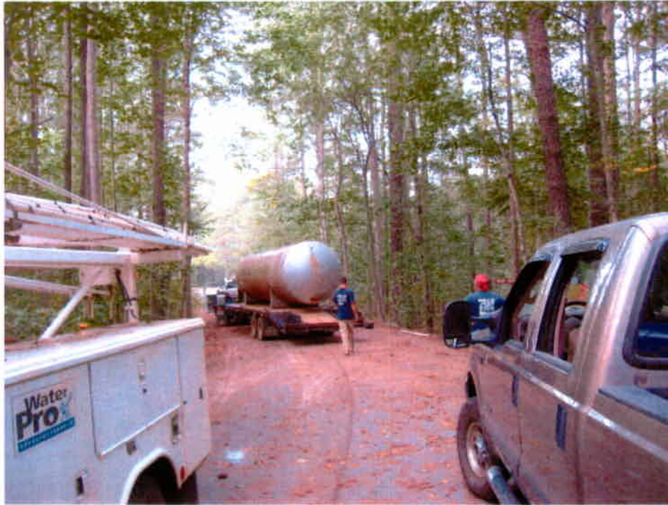
Photograph 7: Transportation of the AST
