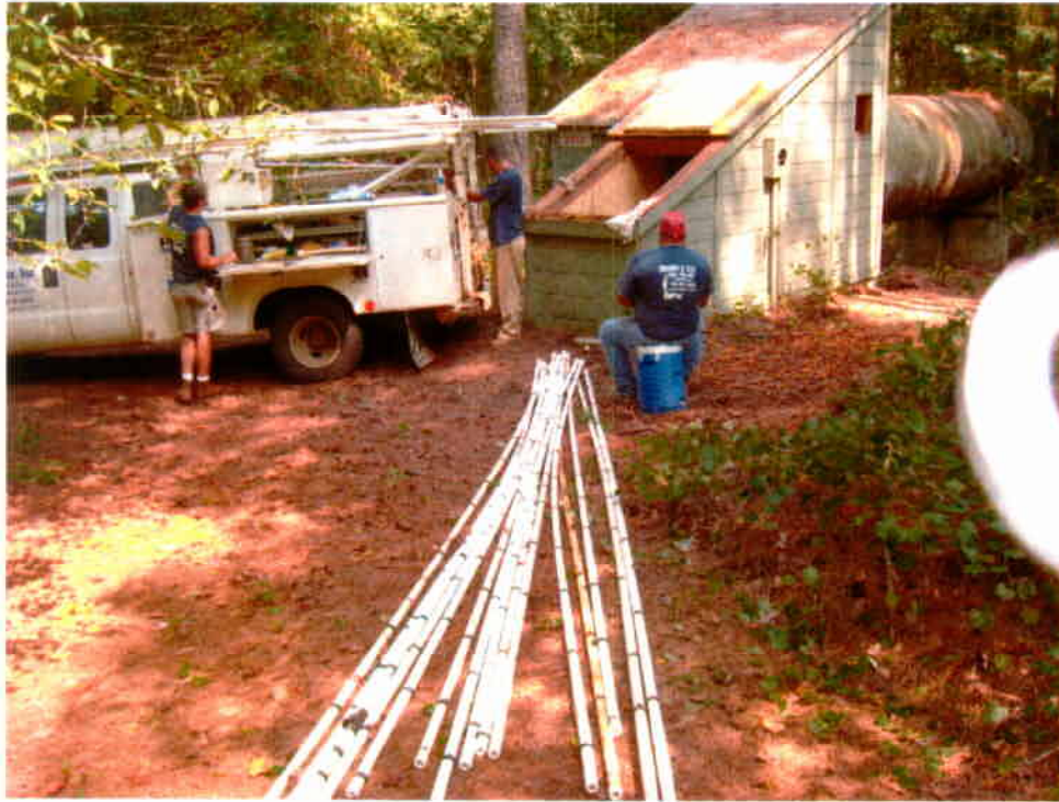
Photograph 3: Removal of 1- inch piping in the well
